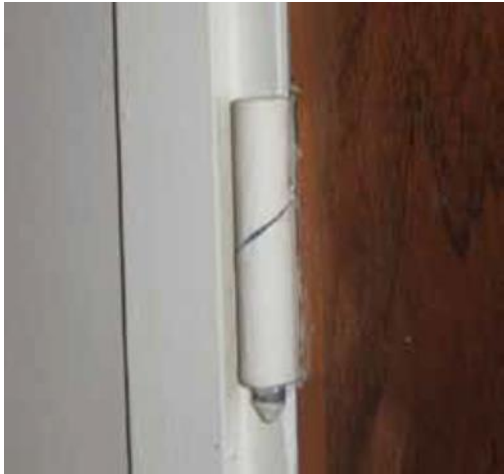
Figure 12 Rising butt hinge
